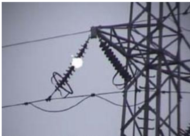
Figure A.28 – Failing external insulation –Example 1
