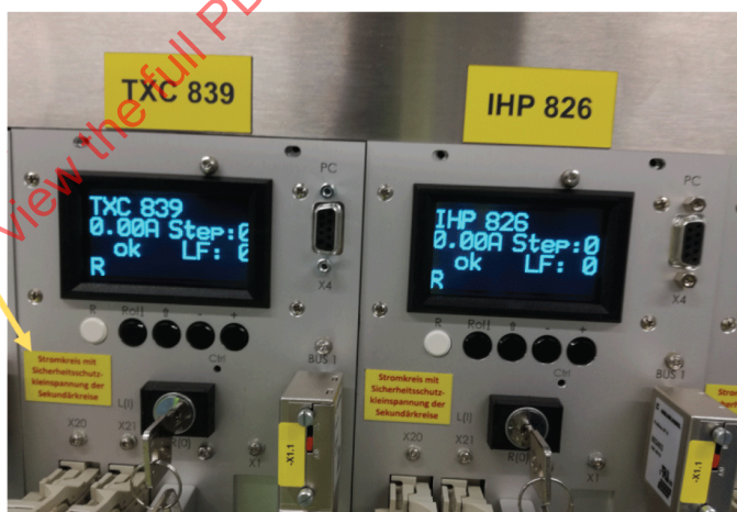
Figure B.6 – Example for field marking (CCRs)
