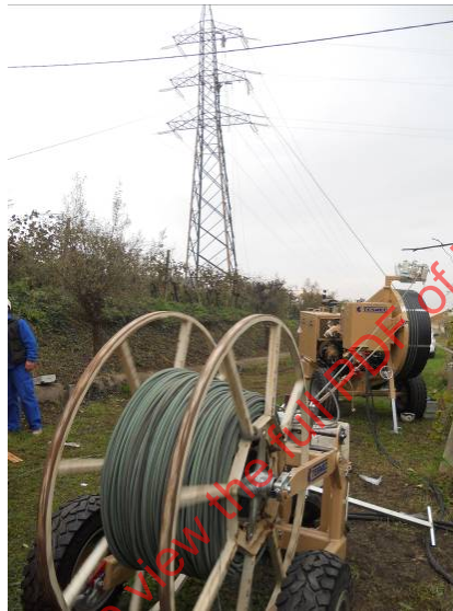
a) Drum puller, two single drums (IEC 60743)
