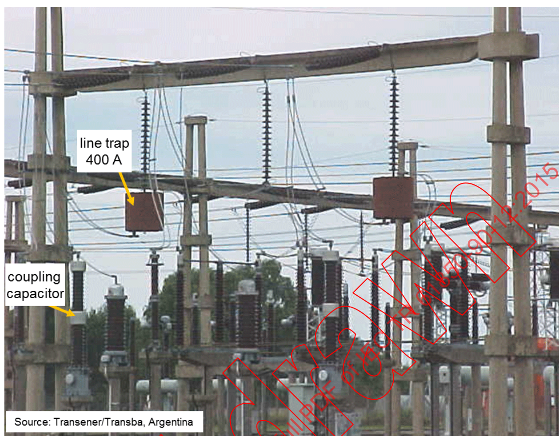
Figure 29 – Phase-to-phase signal coupling
