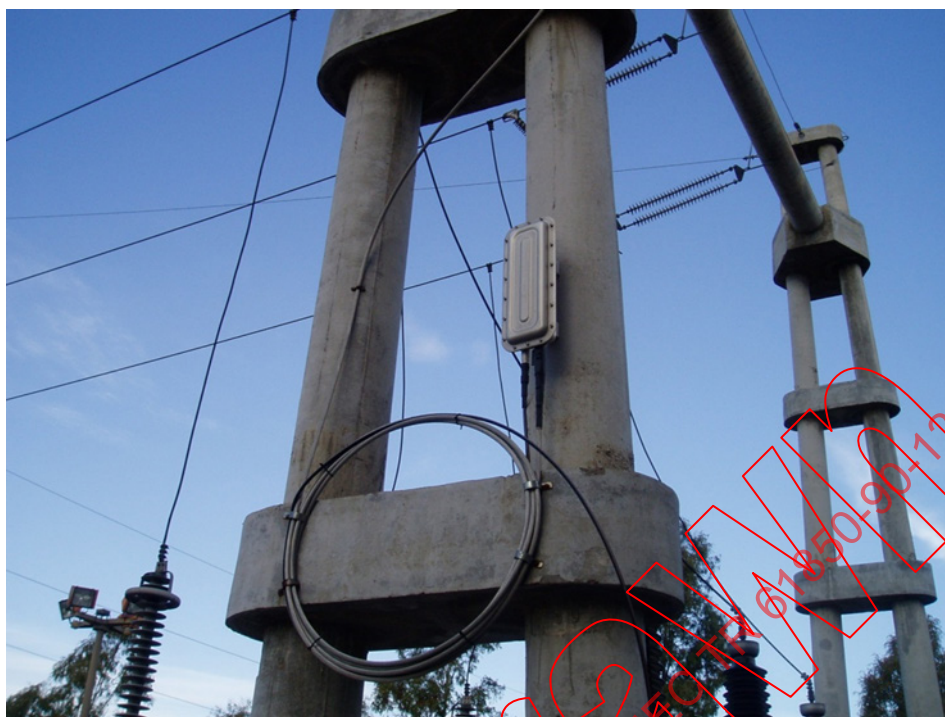
Figure 35 – ADSS installation with splicing box
