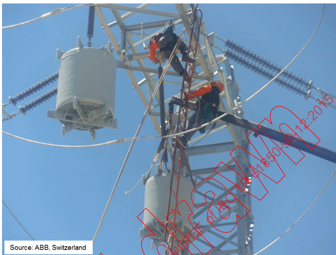
Figure 30 – Power line carrier, line traps
