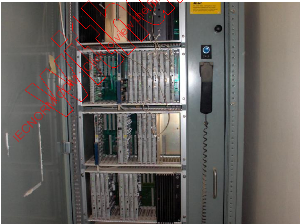
Figure 4 – Cabinet of the substation edge node
