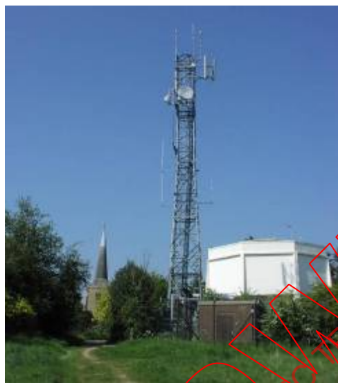
Figure 2.2 Photograph of tower and immediate surrounds
