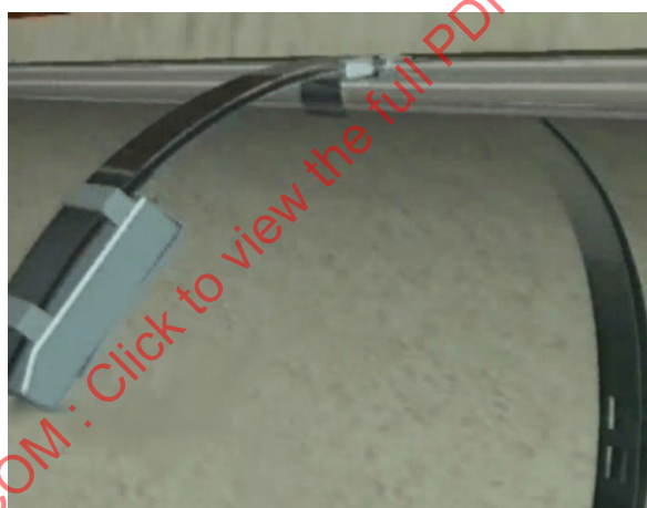
Figure 17 – Spring loaded stainless-steel ring – Conduit fastening
