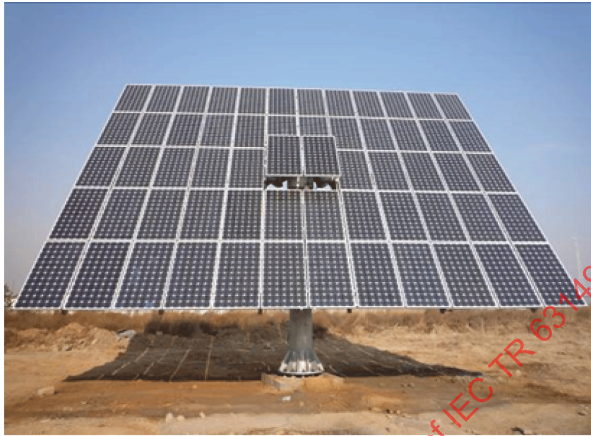
Figure 23 – Double axis-tracking in ground horizontal coordinates
