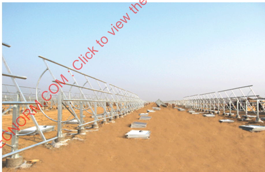
Figure 10 – Manual adjusted supporting structure
