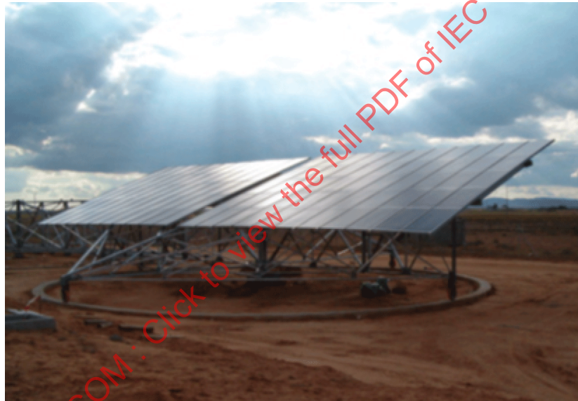
Figure 25 – Solar azimuth tracking (fixed PV tilt)
