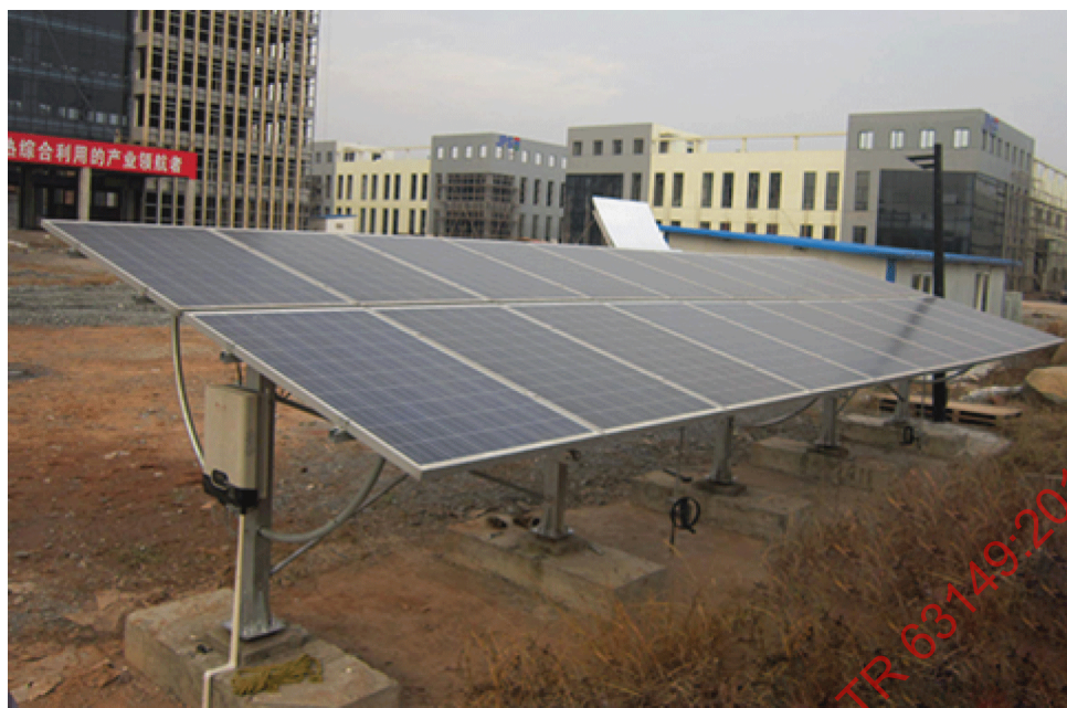
Figure 11 – Manual adjusted PV array
