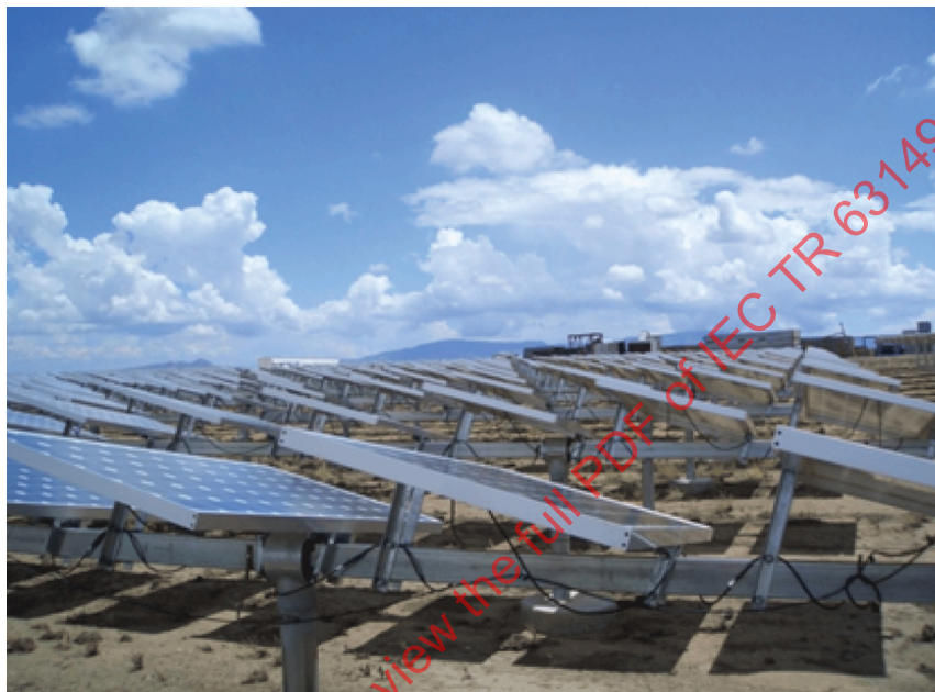
Figure 19 – Tilted E-W tracking (horizontal main axis)
