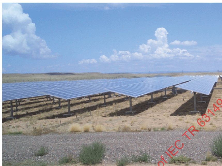
Figure 14 – Horizontal E-W tracking
