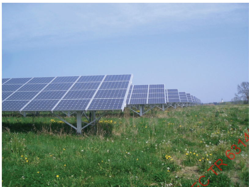
Figure 7 – Fixed PV array on flat land
