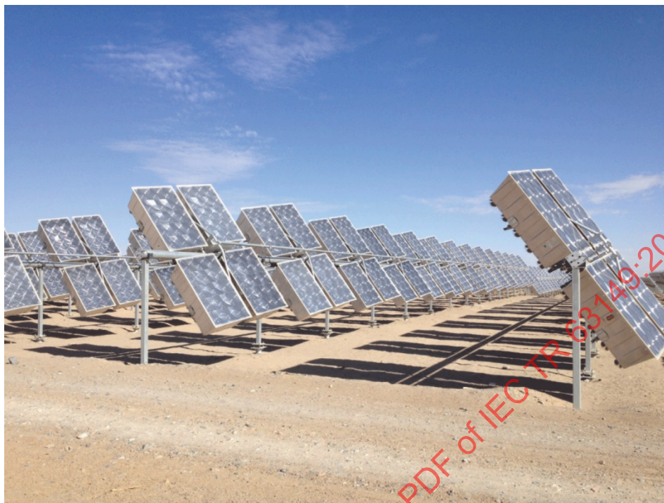
Figure 17 – Double tracking systems (hour-angle and solar declination)
