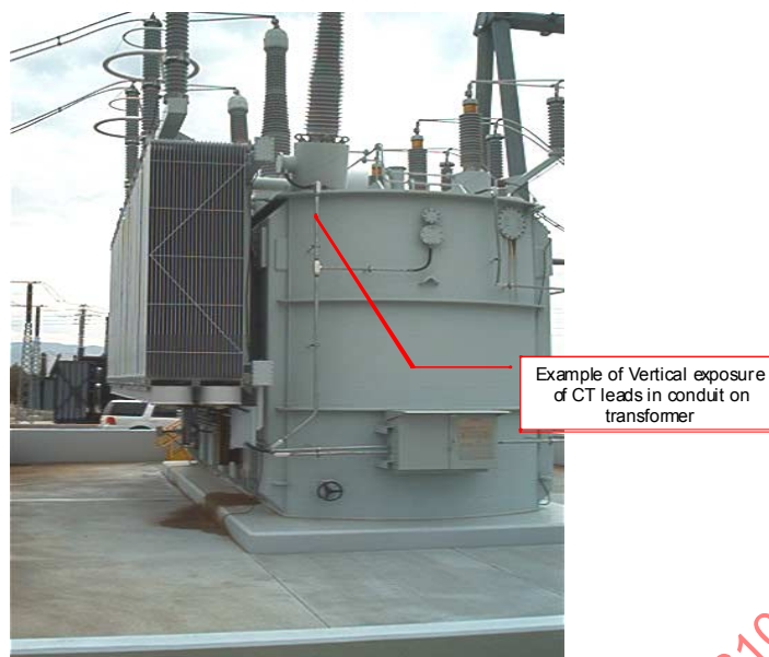
Figure 5 – Vertical conduit geometry for a current transformer (CT)
