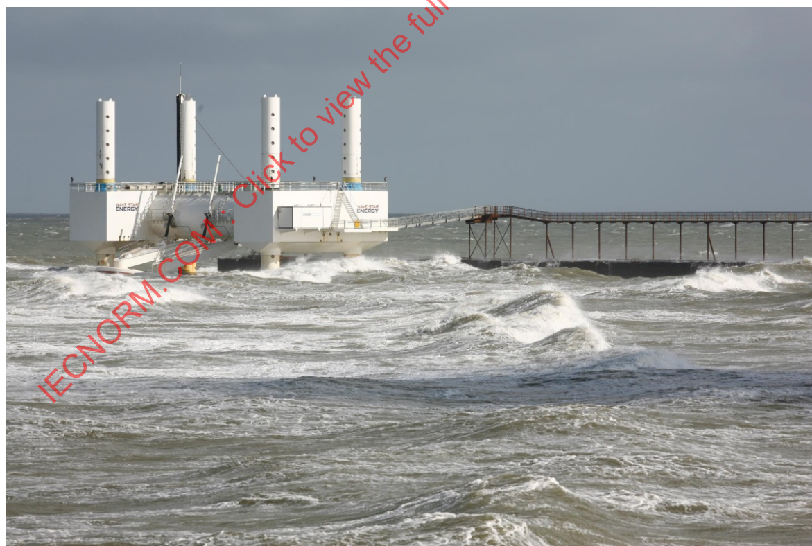
Figure A.1 – The Wavestar prototype (diameter of each float is 5 m)
