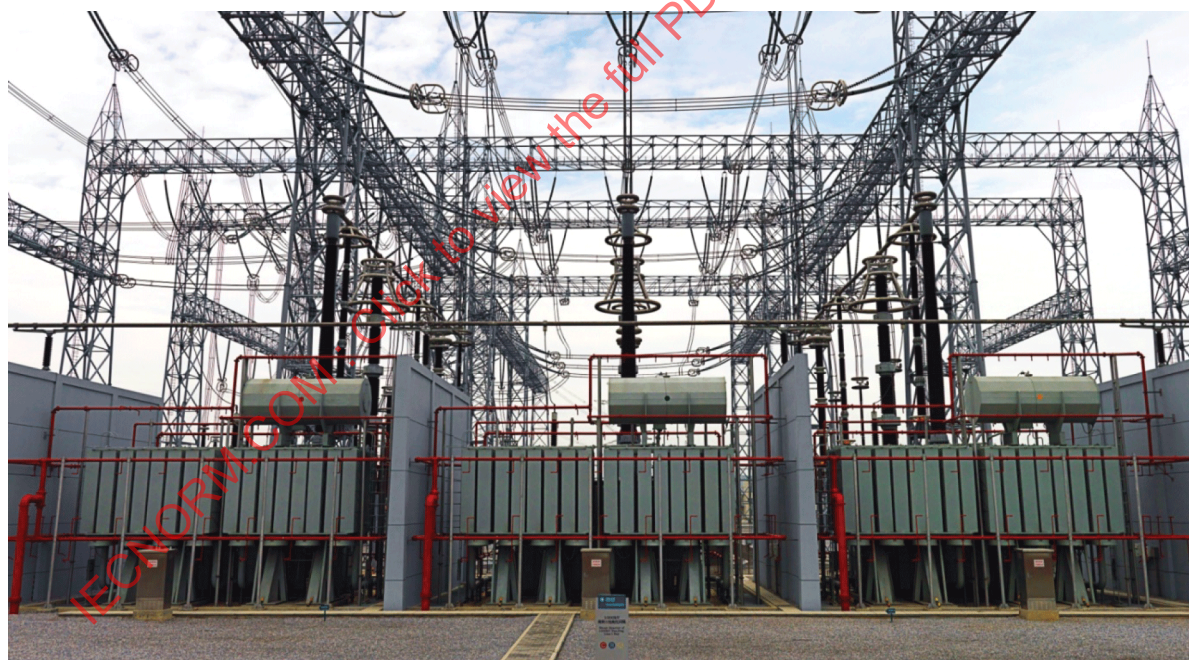
Figure C.2 – UHV AC shunt reactor
