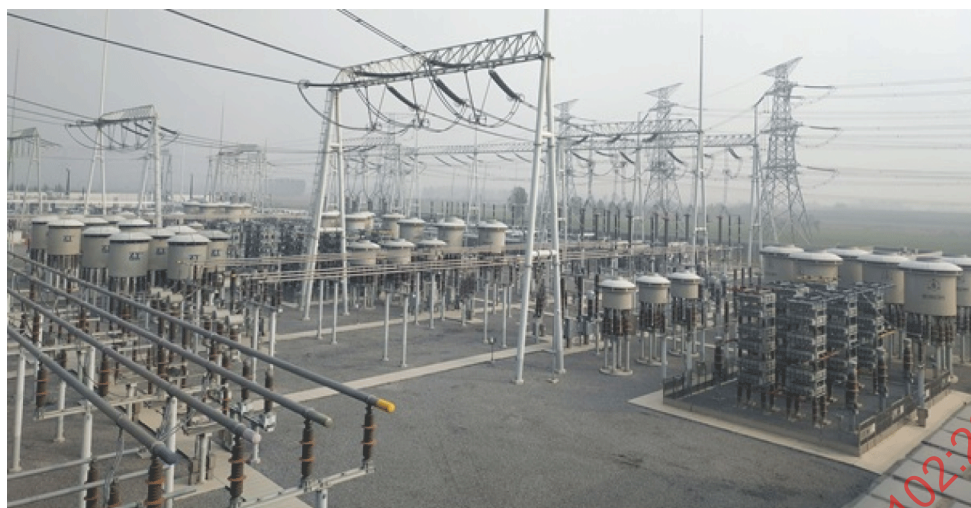
Figure C.3 – Reactor and capacitor at tertiary side of UHV transformer
