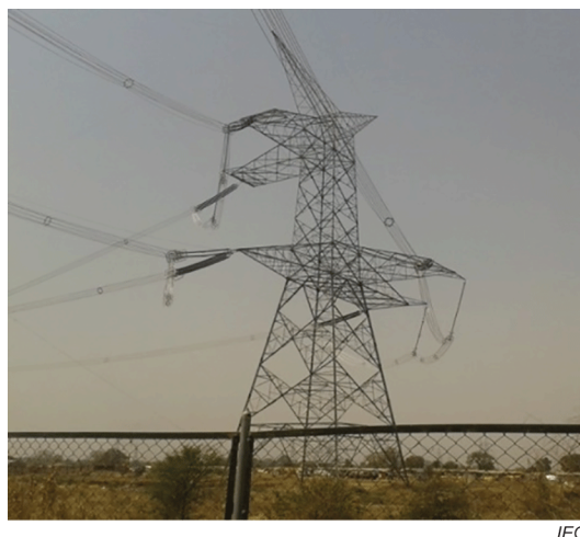
Figure 7 – 1 200 kV single circuit vertical configuration tower
