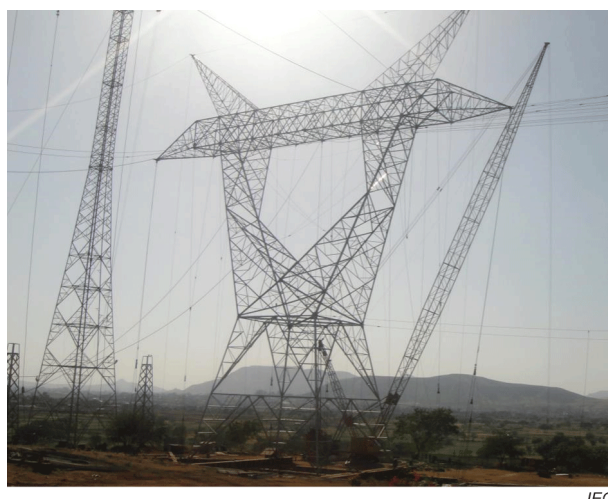
Figure B.8 – 1 200 kV Tower Prototype Testing
