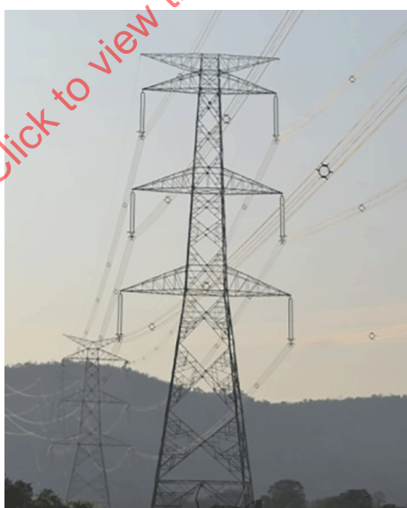
Figure 2 – Typical double circuit vertical configuration tower
