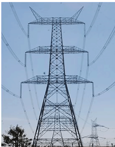
Figure 9 – 1 200 kV double circuit vertical Configuration tower
