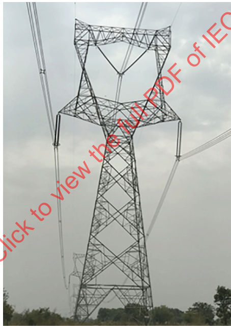
Figure 4 – Typical single circuit delta configuration tower
