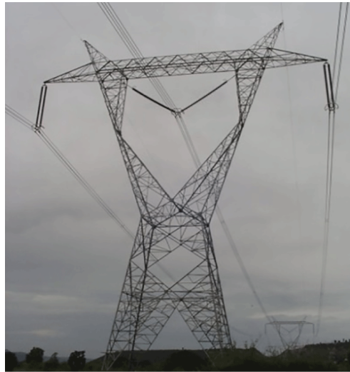
Figure 3 – Typical single circuit horizontal configuration tower
