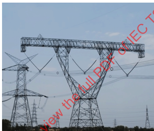
Figure 7 – 1 200 kV single circuit vertical configuration tower
