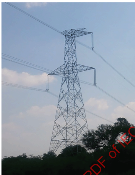
Figure 1 – Typical single circuit vertical configuration tower
