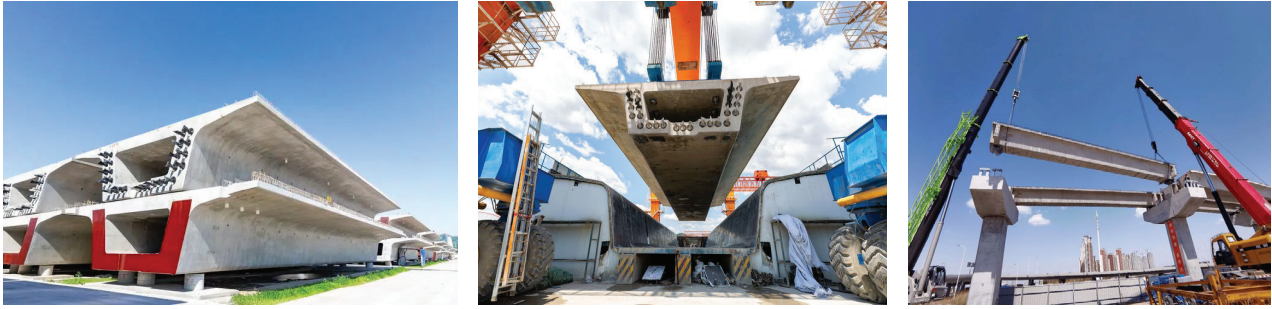
Figure A.12 — Example of a prefabricated bridge
