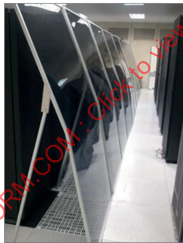
Figure 3 — Cold-air volume around CRAC equipment
