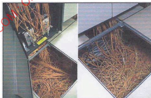
Figure 3 — Example of point-to-point cabling
