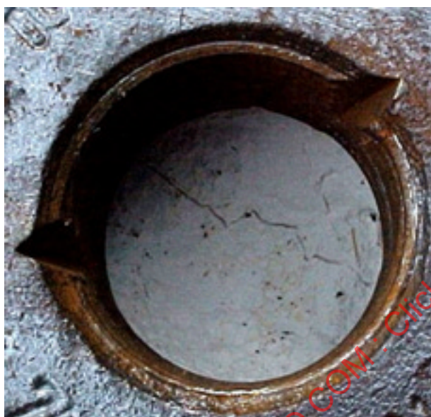
a) Hairline crack without visible sidewalls
