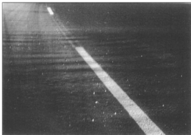
Figure C.9 — Megatexture caused by functioning of finisher
