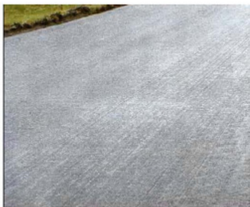
Figure C.4 — Finely milled surface ready for the application of new asphalt concrete top layer (wearing course)
