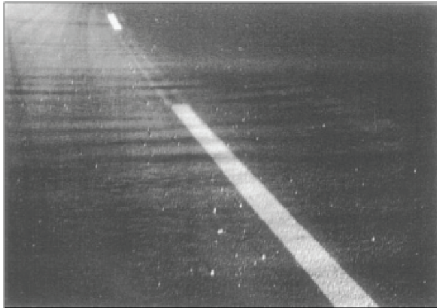
Figure C.9 — Megatexture caused by functioning of finisher
