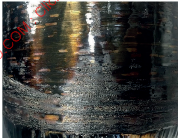
b) Example of Level 3 fire damage
