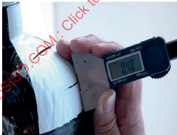
a) Example of Level 1 damage from cuts — Superficial cut and showing device for cut depth measurement
