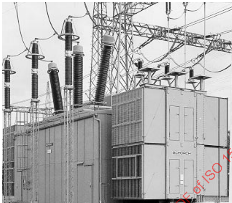
Figure B.3 — Outdoor transformer in enclosure
