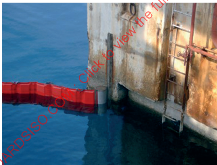
Figure 9 — Example of tidal compensator — View looking down from pier
