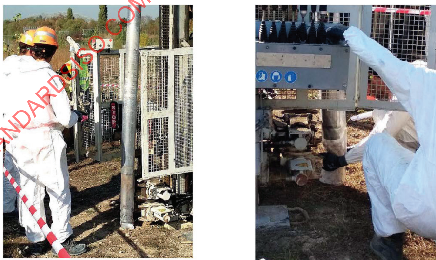
Figure 6 — Sonic drilling
