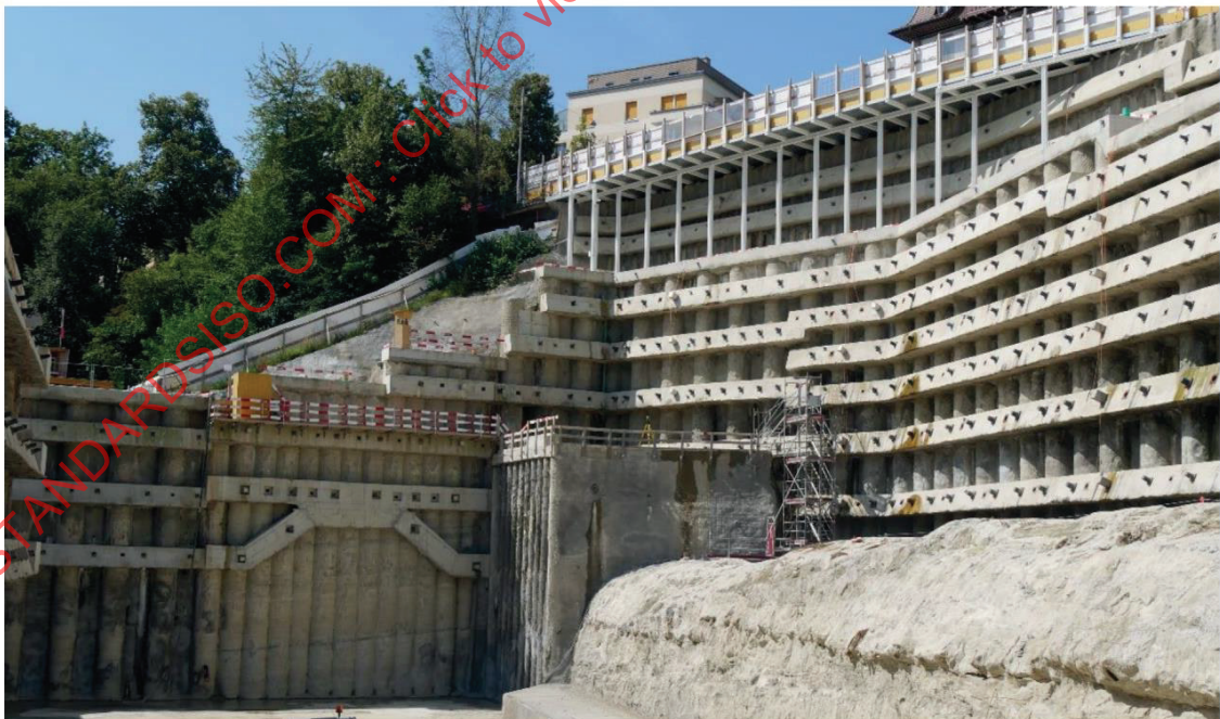
Figure B.8 — Southern part of the excavation with the portal area of the new tunnel in centre and existing tunnel with the lining exposed
