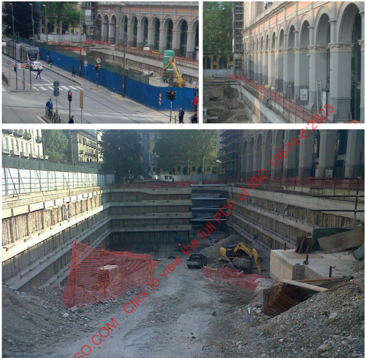
Figure B.1 — View of the working site (Top right: The Porta Nuova Station; top left: road with tram tracks)
