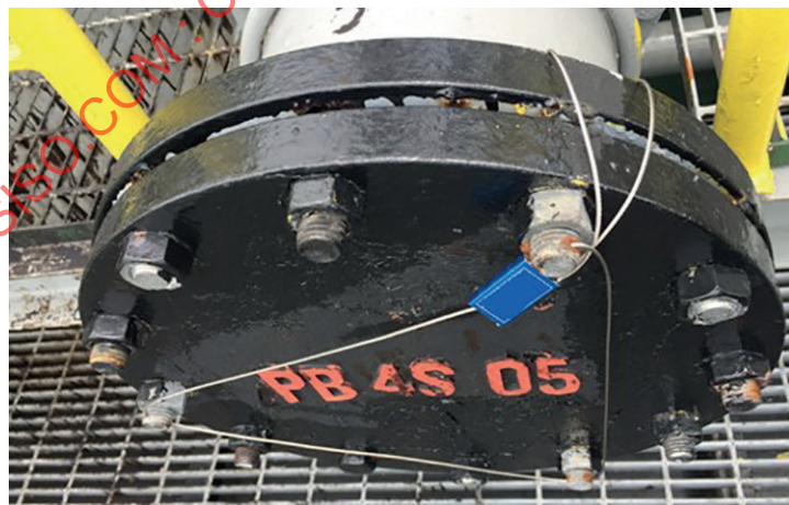
Figure E.2 — Example of sealed pipe blank
