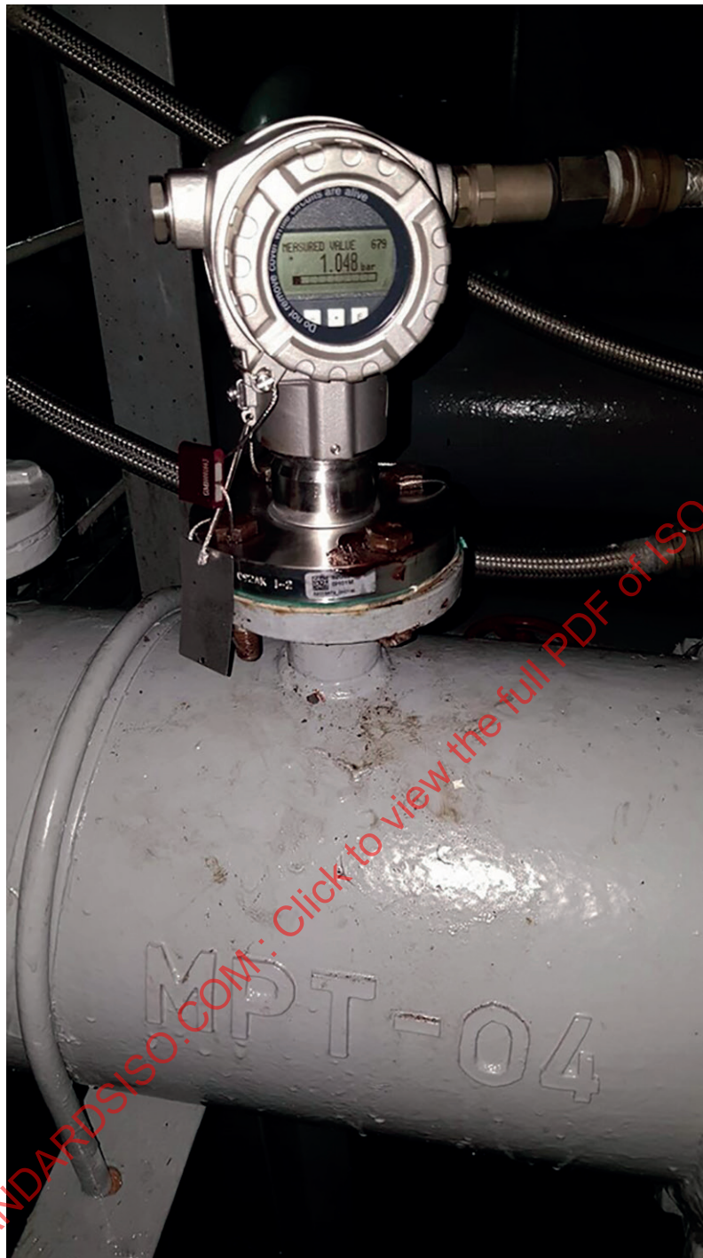
Figure E.3 — Example of sealed pressure transmitter
