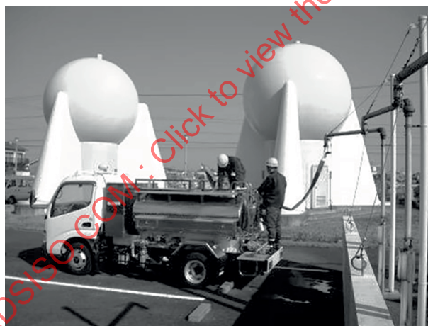
Figure B.4 — Earthquake-resistant static tank
