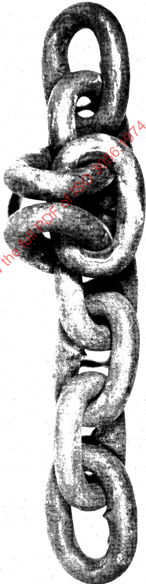
FIGURE 7 — Visual inspection for wear
