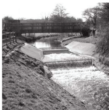
a) Rectangular-throated flume b) Trapezoidal-throated flume
