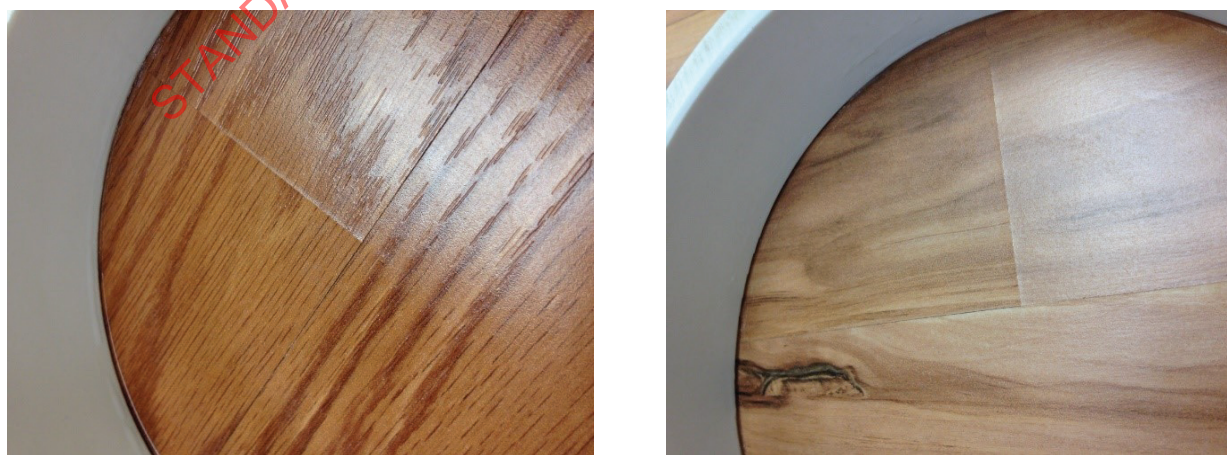
Figure B.2 — Example of slight swelling, small ridge along one or more joints
