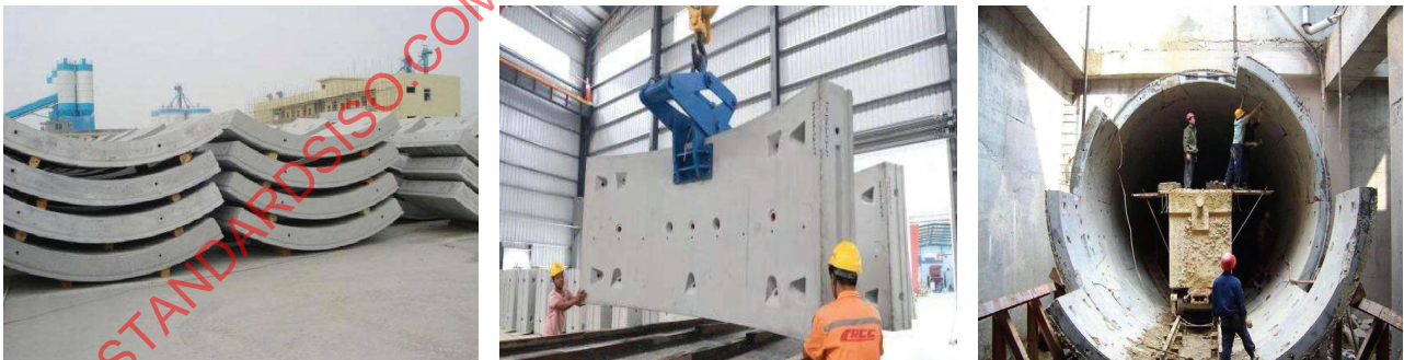
Figure A.14 — Example of reinforced concrete segment
