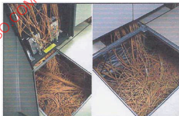
Figure 3 — Example of point-to-point cabling
