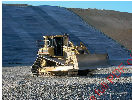
Figure 2 — Placement of drainage aggregate
