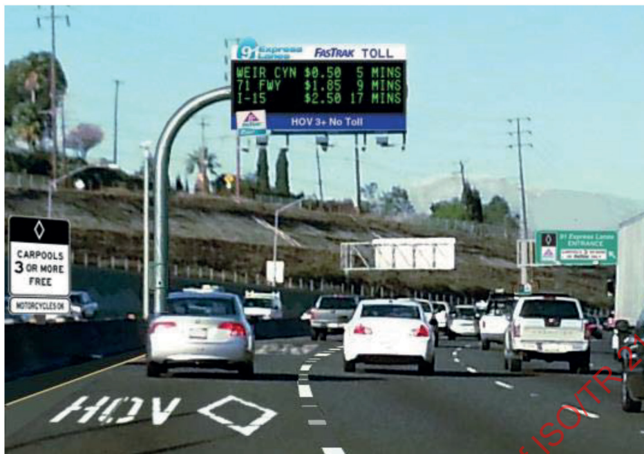
Figure B.4 — Tariff and driving time on message sign (I-91 Express lane in USA)
