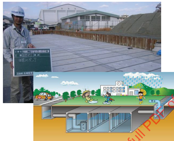
Figure A.39 — Underground stormwater reservoir
