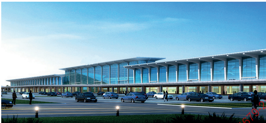
Figure 1 — View of the terminal building
