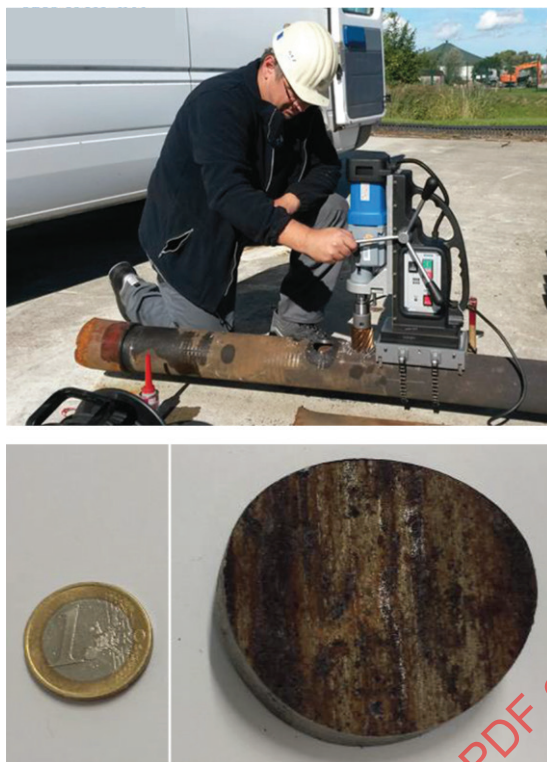
Figure 7 — Cutting out samples of the casing for corrosion inspection (top) - zoomed view of a sample (bottom) (Photos: GFZ)
