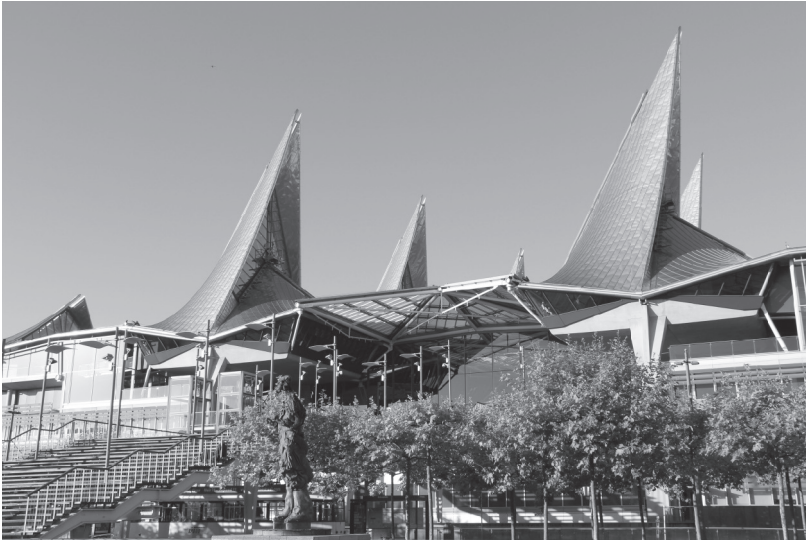
a) Antwerp Court House, Belgium, double skin façade with integrated ventilation system
