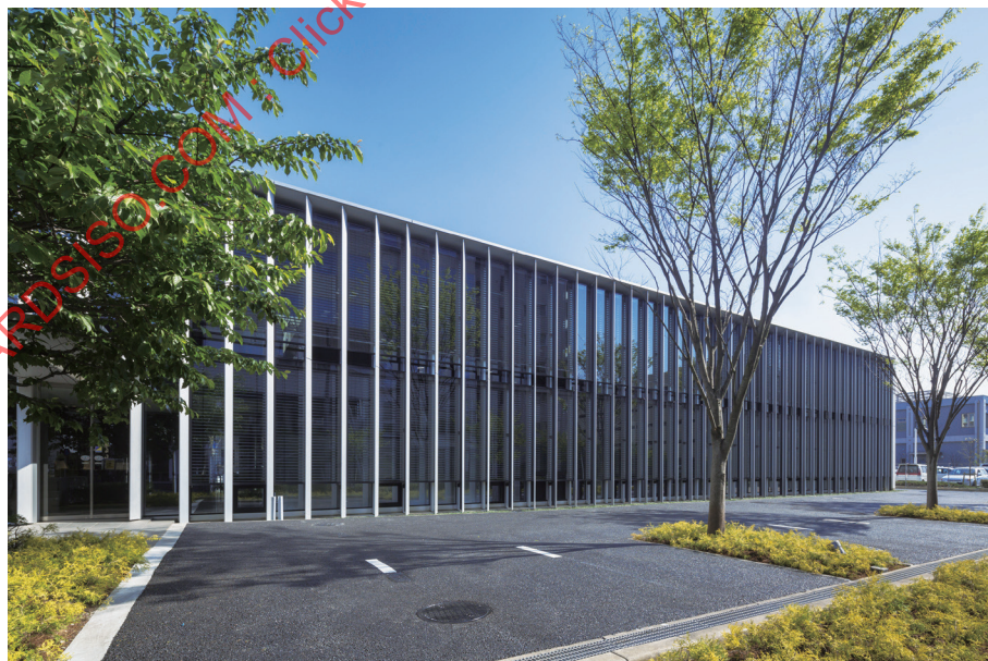
Figure A.2 — Building facade
