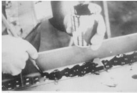
FIGURE 8 - Application of Brushable Sealant
