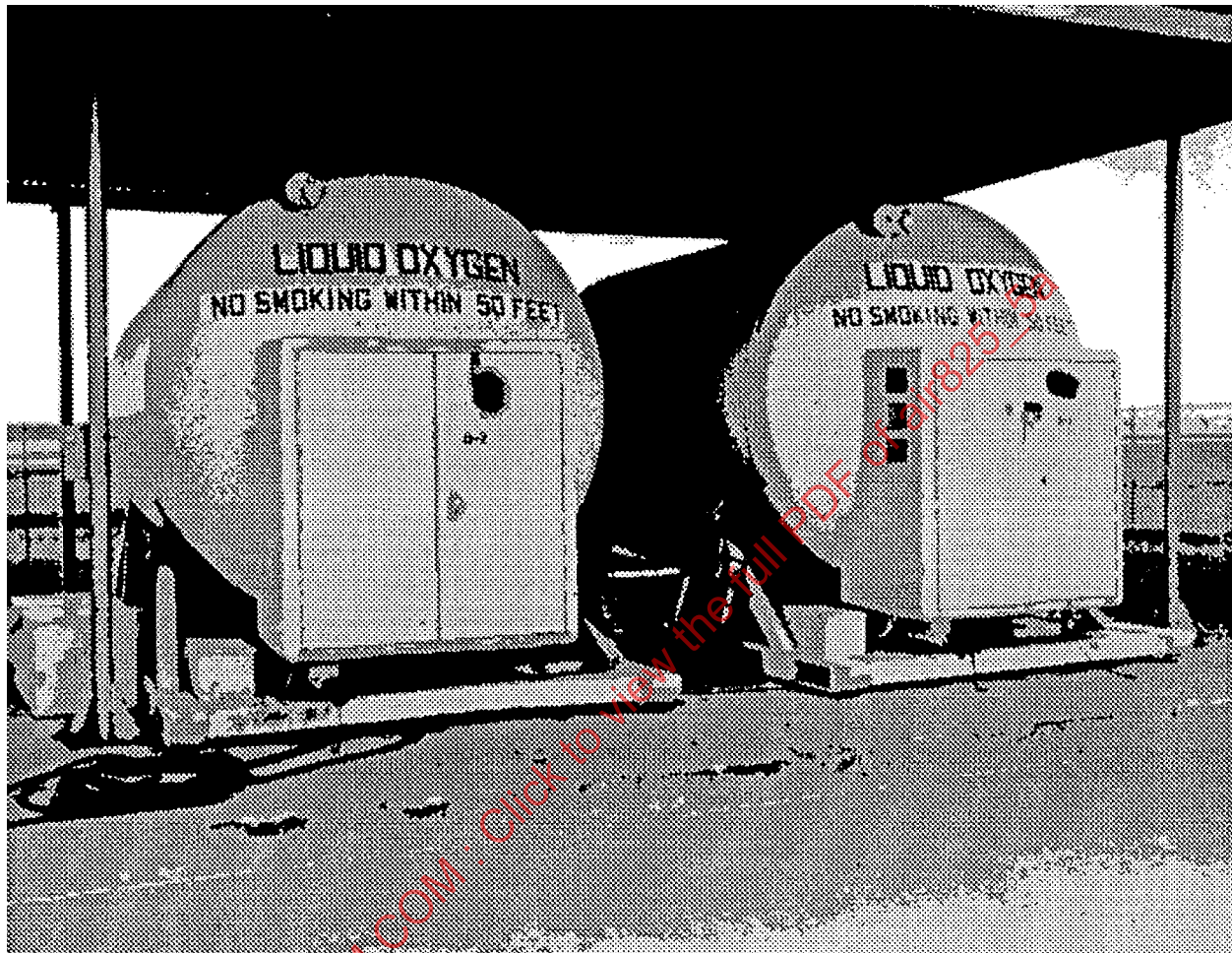
FIGURE 5 - LOX Ground Storage Containers, One Type
