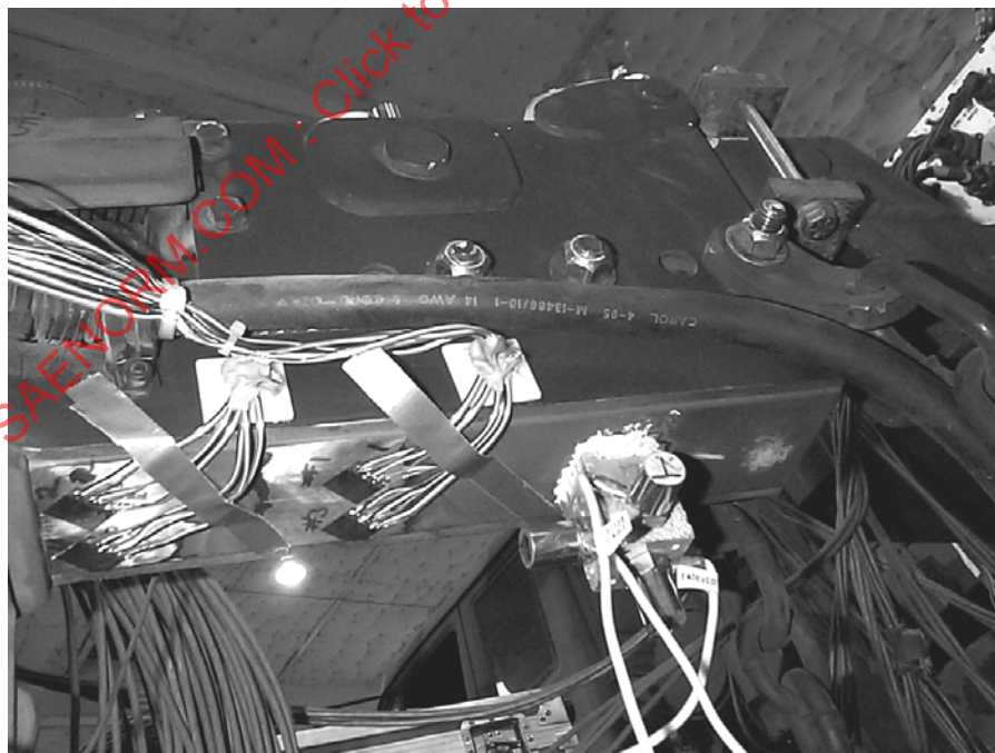
FIGURE 3 - LOCATION AND INSTALLATION OF THE STRAIN GAUGE ROSETTES
