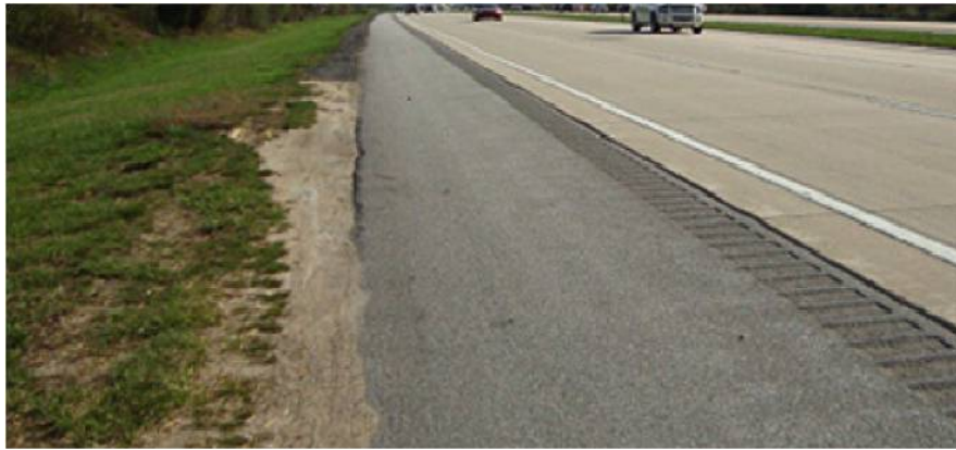
Figure 6 - Example of visually contiguous paved traveled way, a paved shoulder, and a partially usable unpaved shoulder
